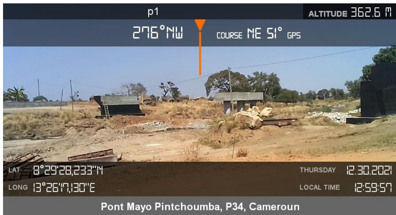
Image 1. Bridge under construction on the Mayo Pintchoumba
