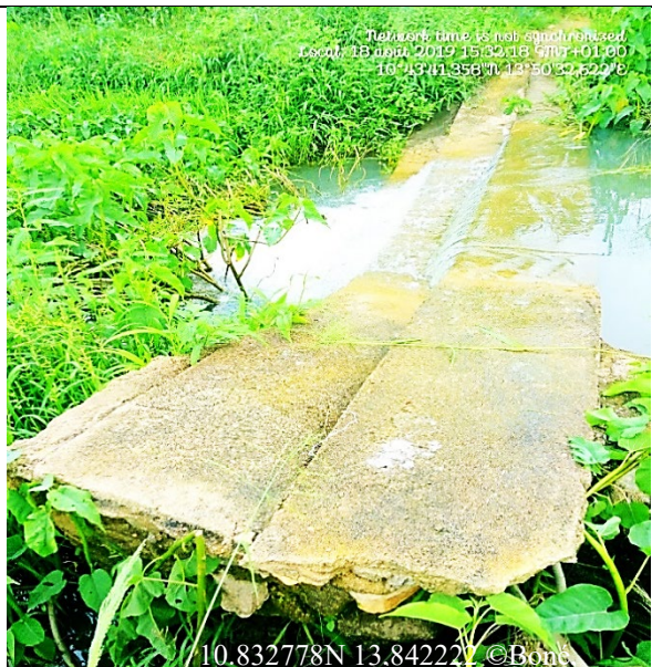
C) Erosion of the protective wings of a masonry forebay at Mandaka (Mokolo)
