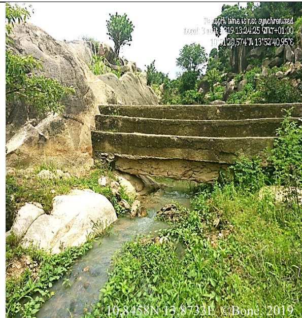
B) Scouring of a concrete forebay at Dzah (Koza)
