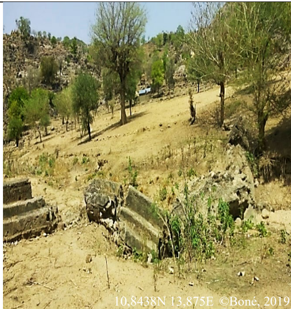
A) Overturning of a masonry forebay at Dzah (Koza)
