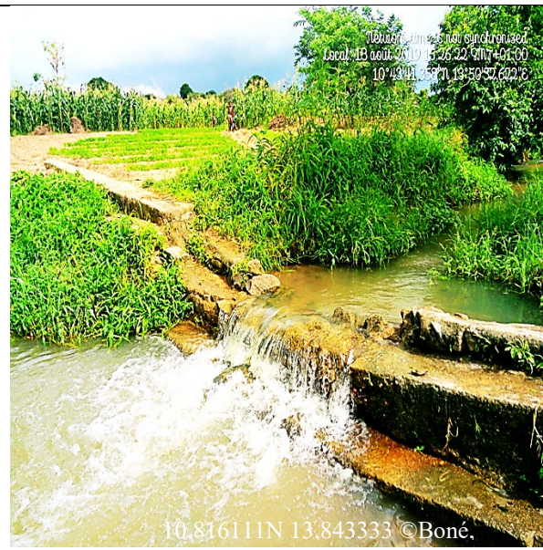
D) Erosion of the retaining wall of a masonry forebay at Mandaka (Mokolo)
